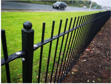
Railing and Gates
