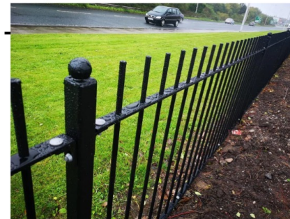
Railing and Gates
