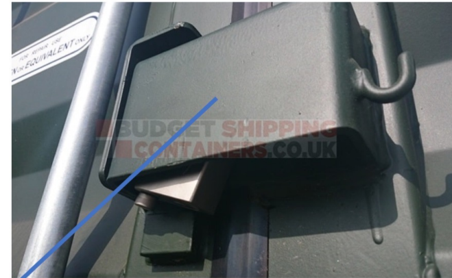
ANTI-TAMPER LOCK BOX (AKA COWL HOUSING) TO CARGO DOORS
