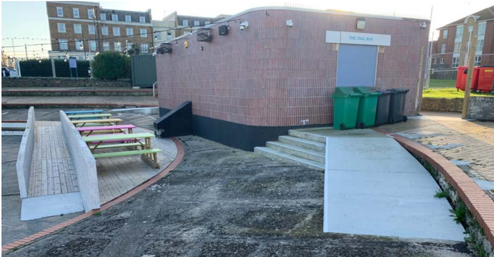
The Oval Pavilion, the café terrace and ramps for accessibility (September 2023).
