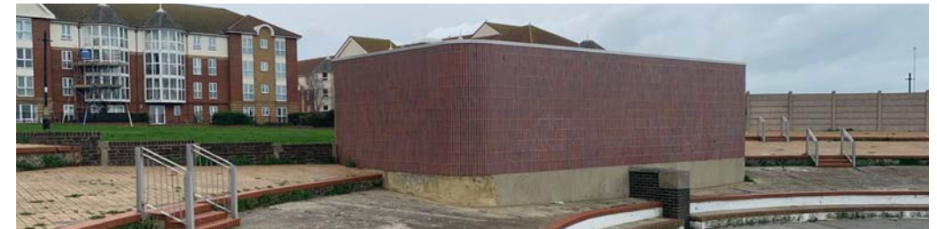
The exterior of the toilet block in July 2021
