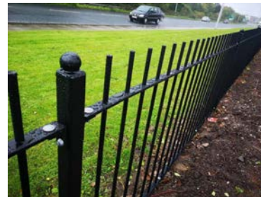
Railing and Gates
