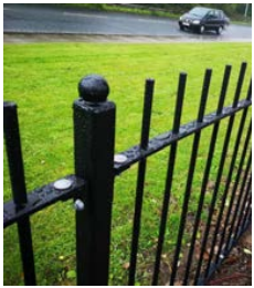
Railing and Gates
