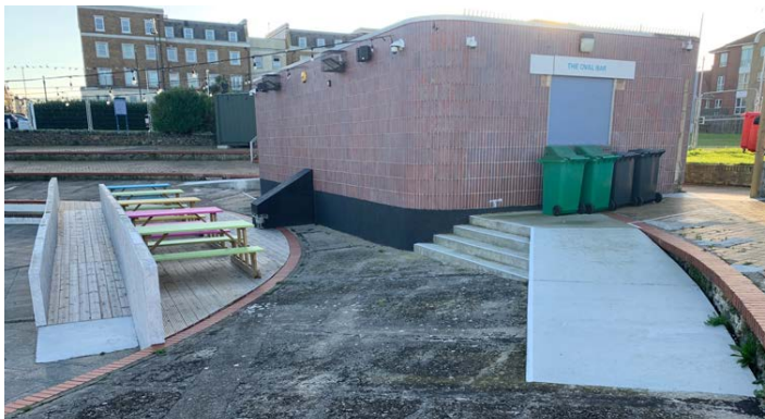
The café terrace, DDA ramps and steps all awaiting handrails
