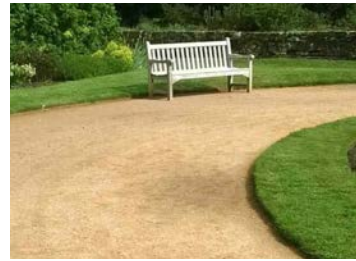
Self-binding compacted gravel path
